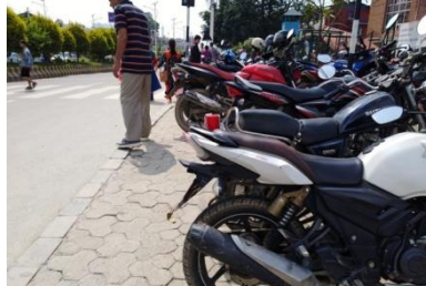
Figure 2: encroachment of footpath by Parking Source: https://encryptedtbn0.gstatic.com/images?q=tbn:ANd9GcSYC8bKUNRZA7YYlvUMDeQhHd2H7EoDxaurlGFZ_uEa-pvGa6FxA
