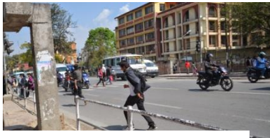
Figure 1: encroachment of footpath by overhead bridge. Source: from internet
